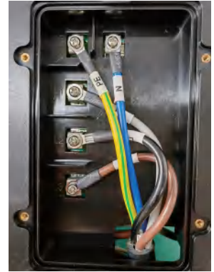
Cable harness diagram FEV-T16/32 (3Ph Connection guide)
