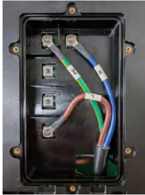
Cable harness diagram FEV-T16/32 (1Ph Connection guide)
